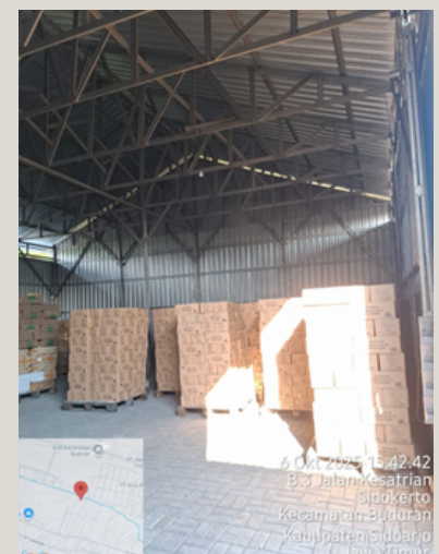
Pict 21. Finished Goods warehouse
